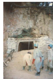
d. Installed support
