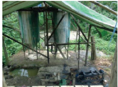
Truss system of tank with conical base
