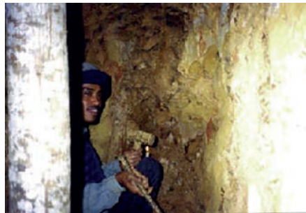
Photo 4.7 Manual Excavation (Do Not Try Without Personal Protective Equipment)
