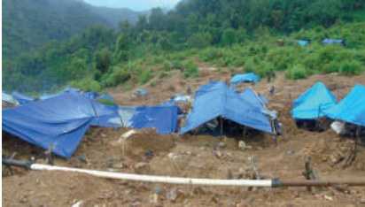
c) Unsafe shafts
