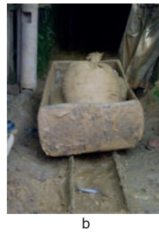
Photo 2.22 Installation of Rails and Bearings a) Steel b) Wood
