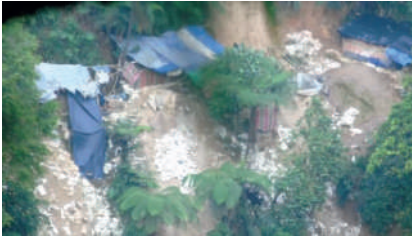
a) Unsafe tunnel entry point
