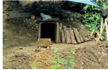
b) Safe tunnel entry point
