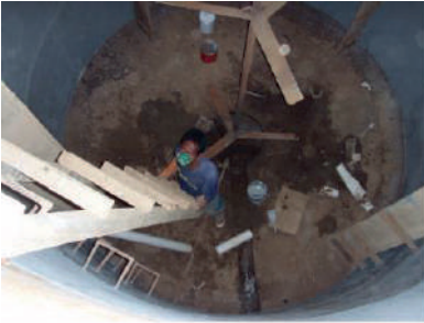
Leaching tank with flat base system
